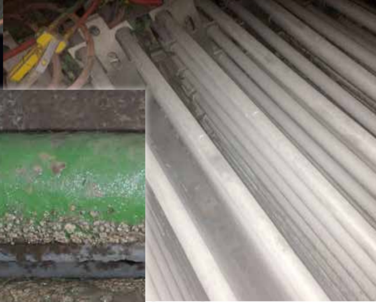
▲ Greenshield inspection in the superheat section after 1 year in service.
