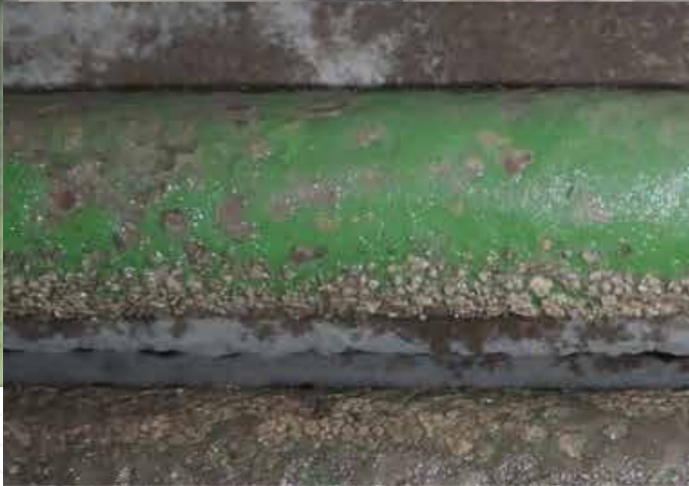
▲ Greenshield inspection in the superheat section after 1 year in service.
