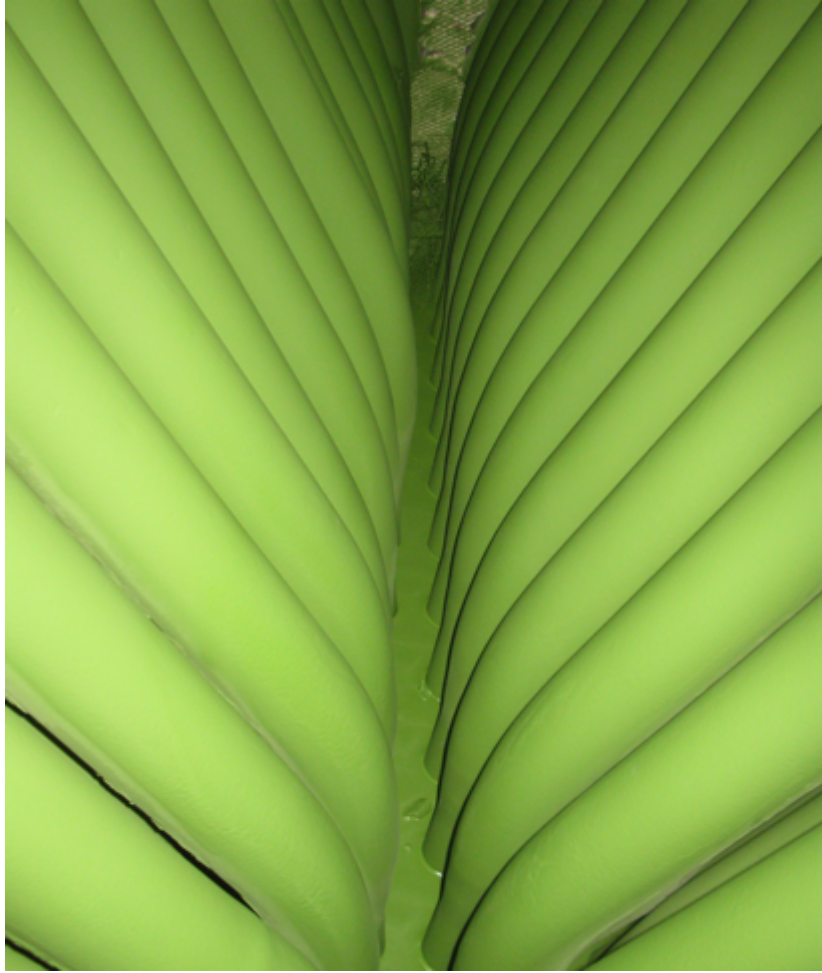
Ceramic coating used to protect hard to reach generating bank mud drum from fly ash erosion damage, Photo by Furnace Mineral Products Inc.
