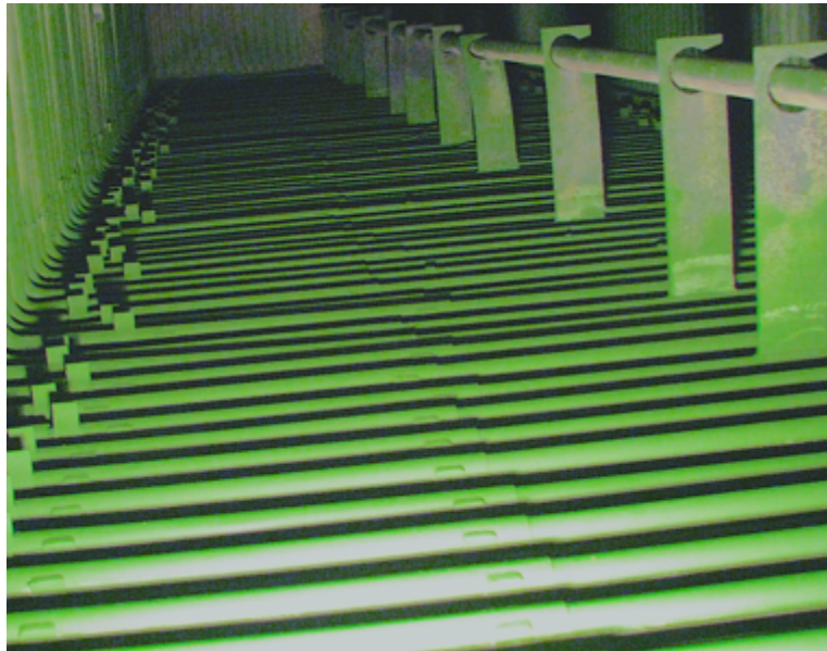
Installation of ceramic coating technology designed specifically for corrosion resistance, Photo by Furnace Mineral Products Inc.
