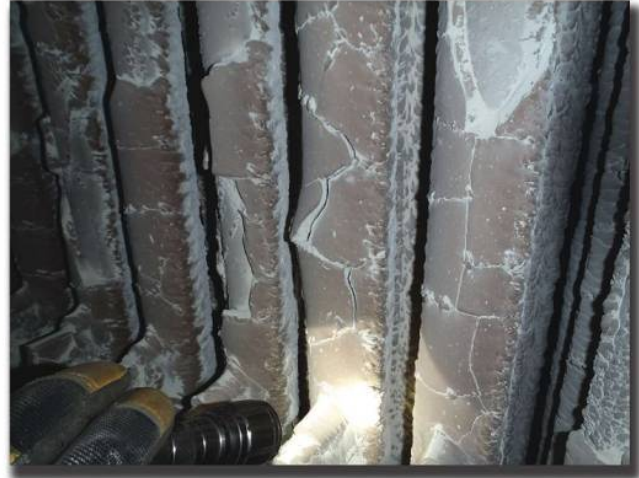
Before being coated, superheater boiler tubes in the Rosebud Operating Services' power plant in Billings experienced severe slag build-up (left) that was removed by sandblasting. After coating the superheater boiler tubes, slag buckles and breaks off (right). Photos courtesy of Dan Gray, Rosebud Operating Services.
