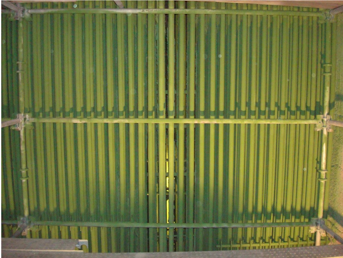
Figure 7: Superheater section at the completion of ceramic coating application
