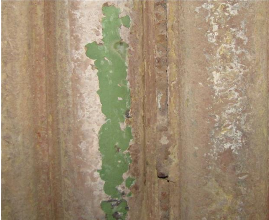
Figure 2: Thin slag deposit removed revealing intact ceramic coating in lower furnace
